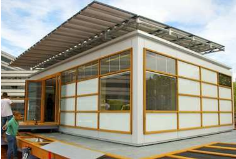
Team NY's Solar Roofpod is a very small dwelling unit, similar in size to that being sought in the adAPT NYC design competition recently launched by Mayor Michael Bloomberg. In addition, these units are equipped with energy collecting devices, water saving systems and food production areas. Sustainability is an integral component of the design.
